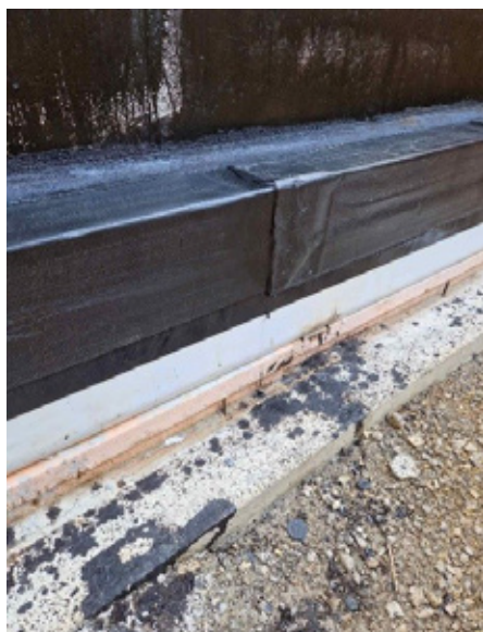
Safety FLEX P se polno navari na LT Bu-tylene Duo R BT
