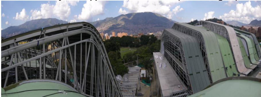
Colombia - Flagon SFC RAL green glued with Flagcol P1M
